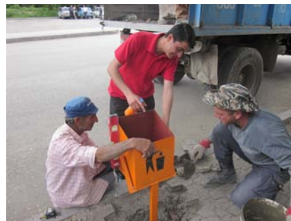
Yeghegnadzor YB members installing trash-bins in the town
